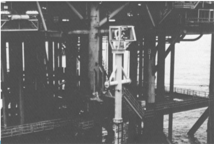
RISER LOWERING ADJACENT TO BRAE 'A'
