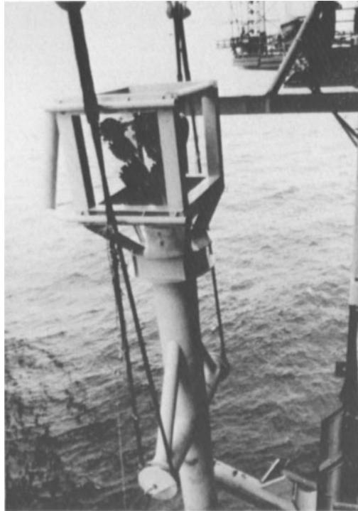
RISER LOWERING INTO DEAD WEIGHT SUPPORT
