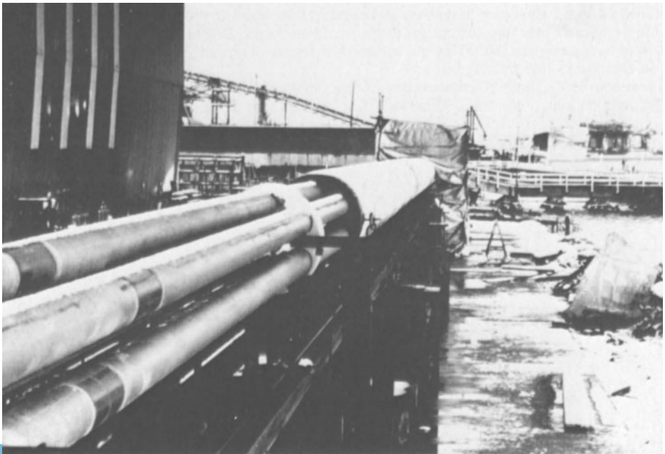
RISER BUNDLE BEING INSERTED INTO CAISSON
